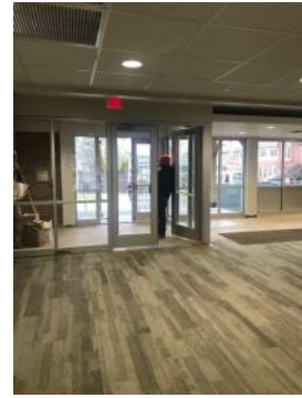
New doors in the Vallette Street entrance.
