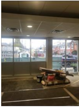
New windows in the Vallette Street entrance.
