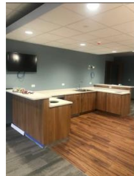
The coffee bar is nearing completion!
