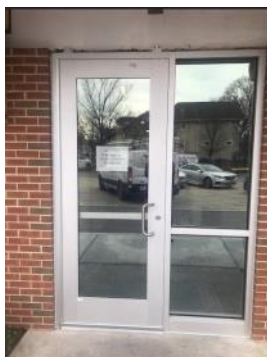
New doors installed at the ACC entrance.
